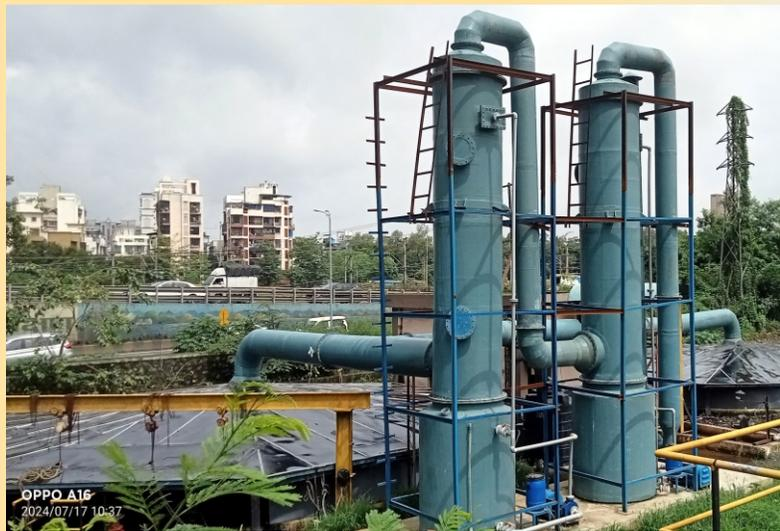
▶ Two Stage Scrubber System. Capacity 5000 CFM.
